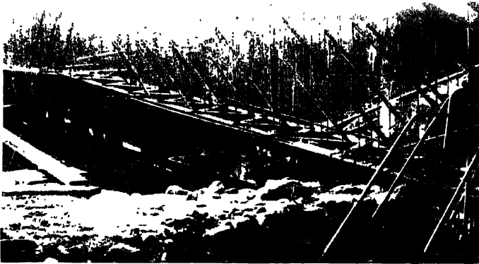
Fig. 291.—Rear Arm of Cantilever : Splice Bars for Hinge on Right.
